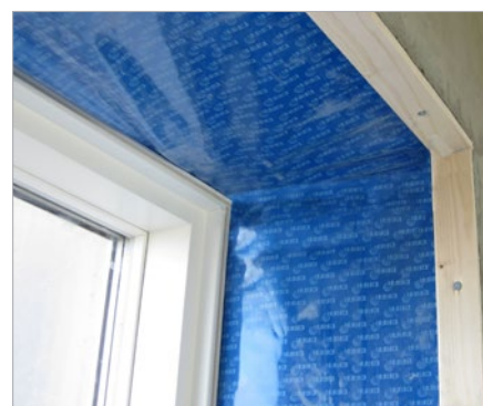
DAFA PE lining foil is CE-marked according to EN 13984
