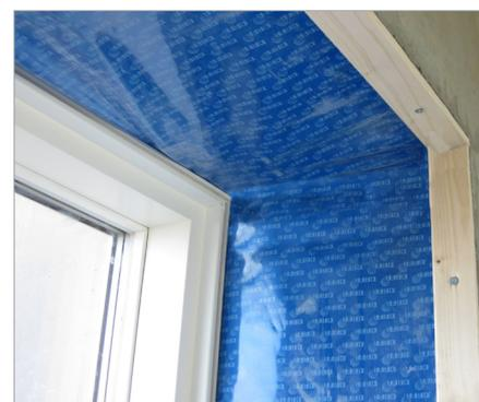
DAFA PE lining foil is CE-marked according to EN 13984
