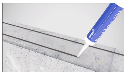
Sealing against plinth / foundation.
