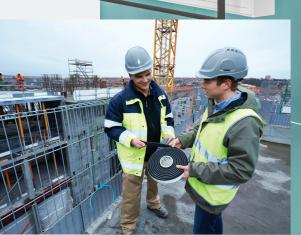
UV tape for facades - highly adhesive UV tape for facades, etc EPDM profiles - seal between the lightweight facade and spacer strips
