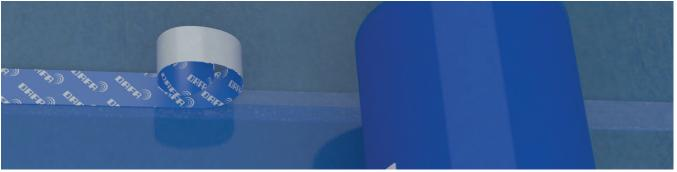
Mount the vapour barrier foil with overlaps and tape with DAFA vapour barrier tape.
