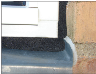
10. After expansion, a completely tight seal will be achieved.
