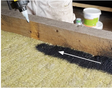
Spray a 10 cm wide first layer lengthwise with the nozzle about 20-25 cm from the surface.
