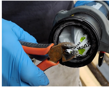
Insert the 600 ml bag of DAFA SprayBarrier into the gun tube and cut the end off using side cutters, just below the metal staple.
