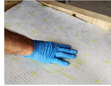
Place the trimmed vapor barrier on top and press it firmly into place. Remember to place the back of the vapor barrier facing downwards.
