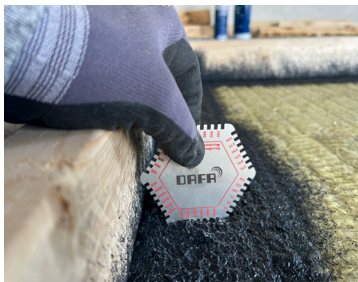
You can use a thickness gauge to ensure the correct layer thickness.
