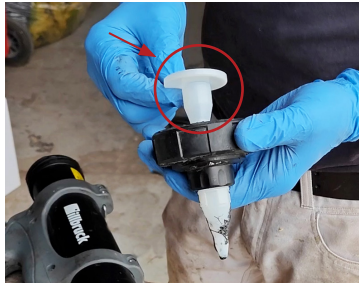
Insert the long caulk nozzle into the small caulk nozzle.
