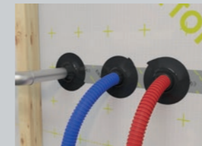
Mounted on vapor barrier
