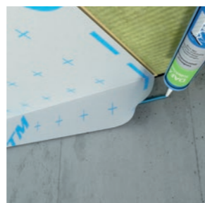
DAFA foil adhesive creates an airtight bond between the vapor barrier and surfaces such as render, concrete or untreated wood.
