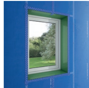
Window frames are easily handled using DAFA lining foil.
