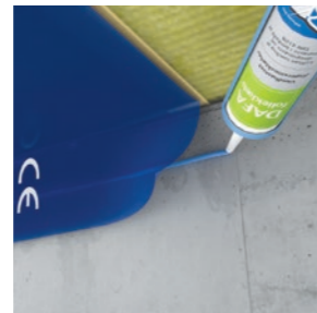
DAFA foil adhesive is used to create a sealed bond between the vapor barrier foil and surfaces such as render, concrete or untreated wood.
